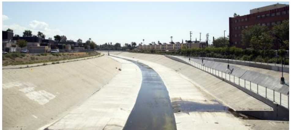
Starting in 1938, the U.S. Army Corps of Engineers channelized the LA River, creating concrete channels for nearly the entire length. Photo: City of Los Angeles River Revitalization
