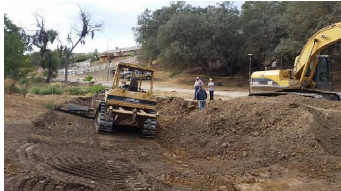
Heavy Equipment doing initial grading. Credit: Upper Salinas - Las Tablas Resource Conservation District.
