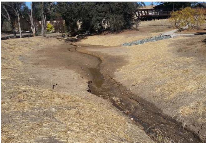
Heavy Equipment doing initial grading. Credit: Upper Salinas - Las Tablas Resource Conservation District.
