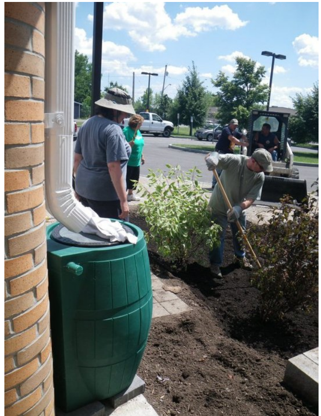
Building a demonstration rain garden.
